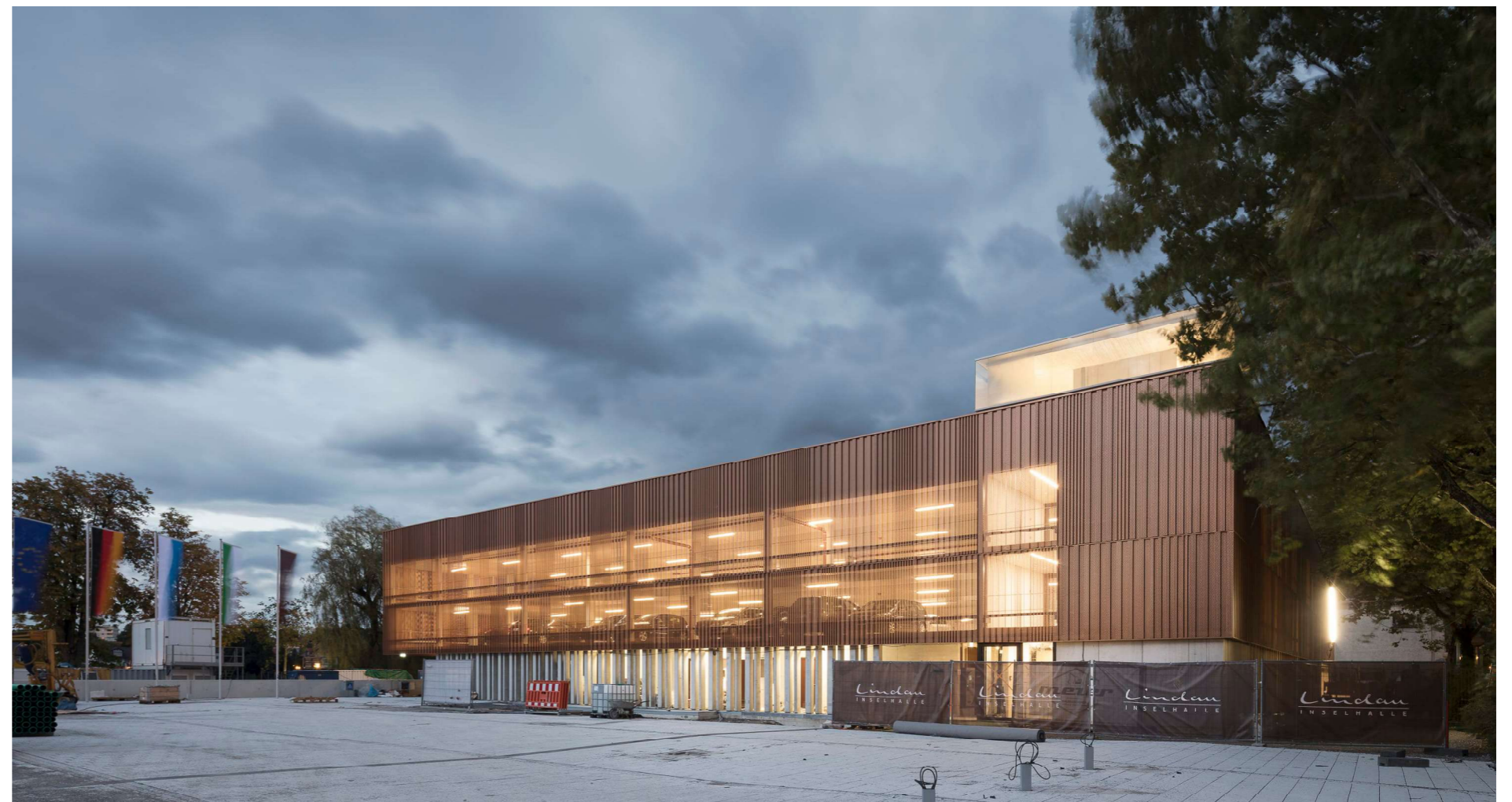
Photograph of Multi-storey Car Park, Lindau, Germany (Architects: Auer + Weber)
